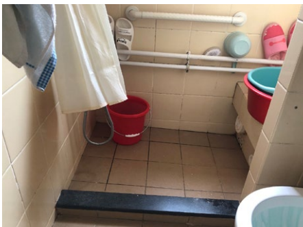
Installation of grab bar
